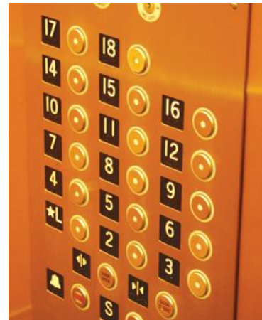
This elevator panel “skips” the thirteenth floor. The floor is not actually missing—the computer that controls the elevator adjusts the floor numbers above 13.
